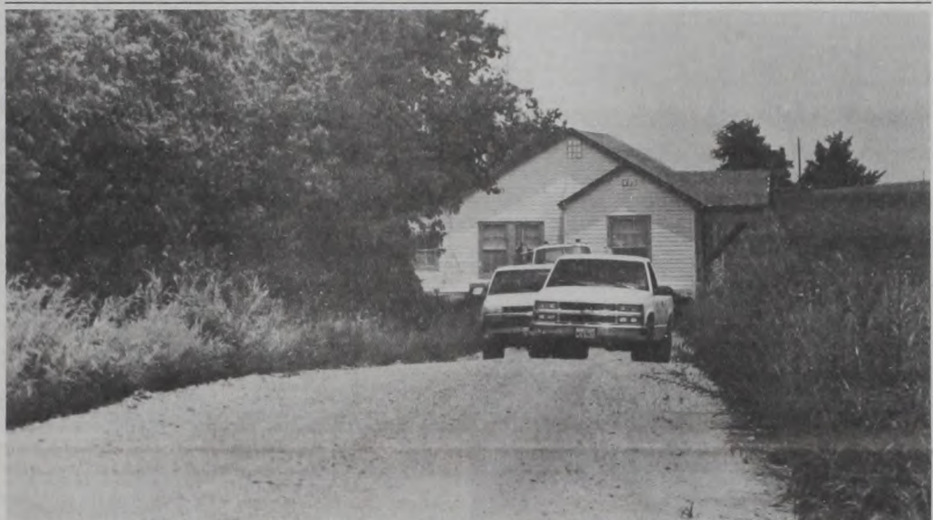
MOVING DAY — House movers ran into several problems Wednesday afternoon moving this house from Zipper Hill. Culverts, narrow roads, and trees hampered the relocation to CR 447. The road remained
