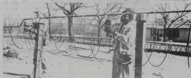
Subcontractors for Phoenix Fabricators, builders of the new 200,000-gallon elevated water storage tank for the City of Muenster, drilled pier holes this week and built reinforced concrete piers three feet wide and 17 feet deep. Eight piers go down to a load-bearing shale formation. The slab foundation for the elevated tank should be finished by Feb. 5. It will include the main service pipe which is 12 inches in diameter. The bottom photo shows steel reinforcement assembly.
