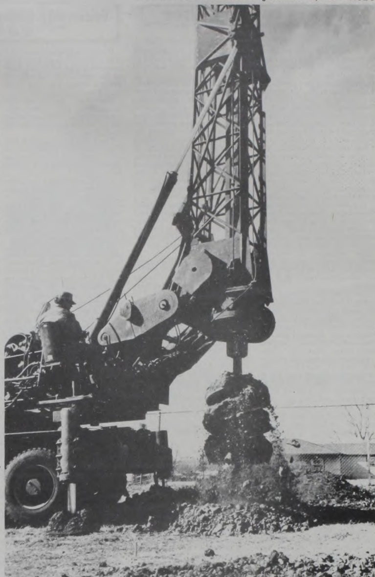
Subcontractors for Phoenix Fabricators, builders of the new 200,000-gallon elevated water storage tank for the City of Muenster, drilled pier holes this week and built reinforced concrete piers three feet wide and 17 feet deep. Eight piers go down to a load-bearing shale formation. The slab foundation for the elevated tank should be finished by Feb. 5. It will include the main service pipe which is 12 inches in diameter. The bottom photo shows steel reinforcement assembly.
