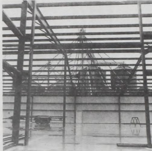
Muenster Milling gets new addition.
