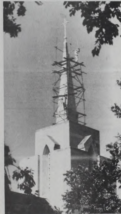
Sacred Heart Church loses cross and section of steeple to repairs.
