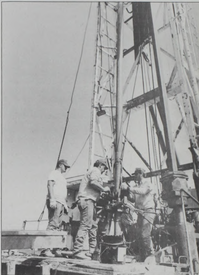
THE CREW OF JIMMY JACK BIFFLE WATER WELL DRILLING COMPANY began drilling Muenster's new city water well Tuesday afternoon and finished the pilot hole Wednesday morning, logging the well at 9 m. The 635-foot-deep well has 48 foot more water sand than the last city well drilled and will pump 150 gallons per minute. The city will now install a 3600-foot trench for the water line from the new well to the supply tank. Working on Biffle's rig Tuesday included, l to r, Brian Huckaby, Herkey Biffle and Cris Aston.
