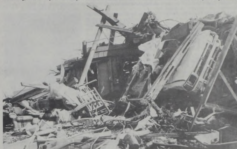
THIS PILE OF RUBBLE is what remained of the Jack Schoppa home Monday morning. Quick response from volunteers helped in the pick-up of salvageable items and the long job of clean-up.
