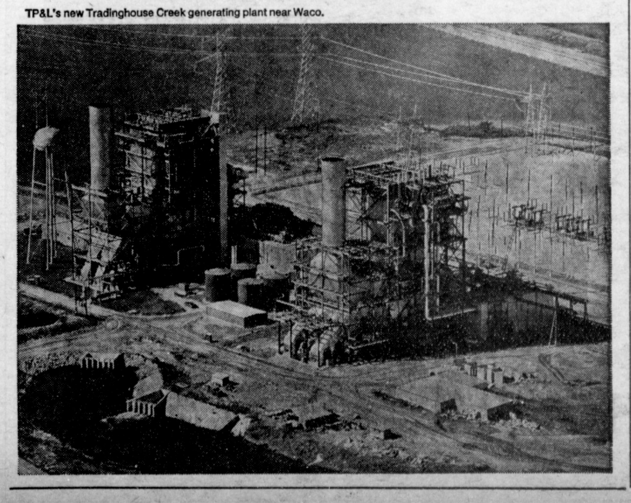
TP&L's new Tradinghouse Creek generating plant near Waco.
