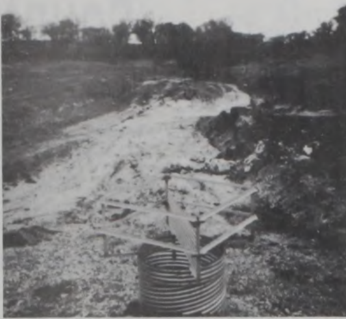
RECENTLY-CONSTRUCTED grade stabilization structure northeast of Muenster. SCS Photo
