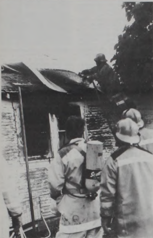
MUENSTER and MYRA FIREFIGHTERS responded to a fire at the Francis Fuhrmann home Tuesday evening, quickly extinguishing the blaze. The fire was confined to the kitchen area with extensive smoke damage throughout the house. Janie Hartman Photo
