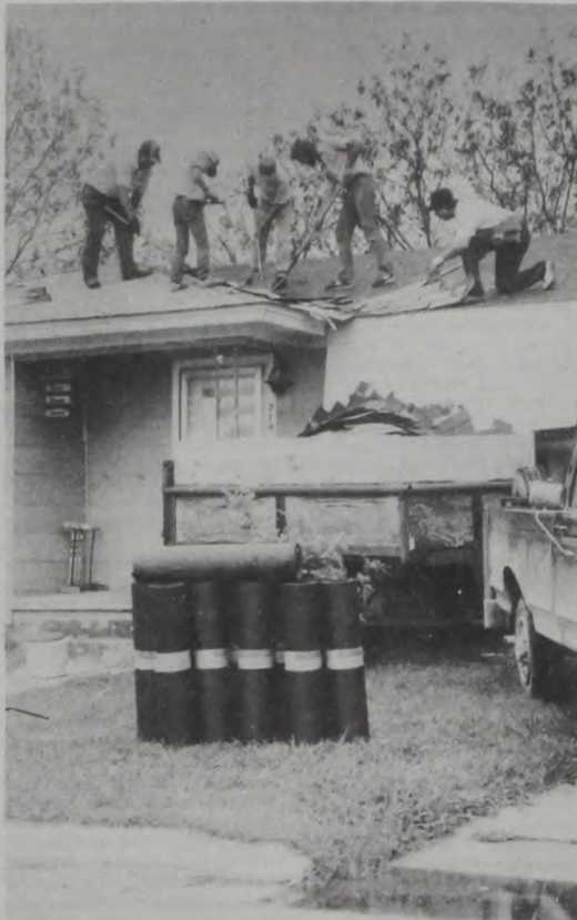
LOCAL ROOFERS have been busy the last weeks repairing dozens of Muenster residents' roofs. The recent heavy rains have delayed the works which went into full swing this week as weather began to cooperate. Workers are shown above removing the damaged tiles from Randy and Ruth Barnhill's home. Janie Hartman Photo
