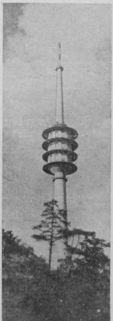
GETS THE MESSAGE—Jutting through the trees, this new 65-foot tower completes telephone message in Berlin, West Germany.
