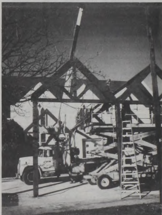
THE ABOVE PHOTO, at right, shows the beginning of construction on the covered protected entry from Sixth Street to the south door of Sacred Heart Church. Photo courtesy Eddie Fleitman
