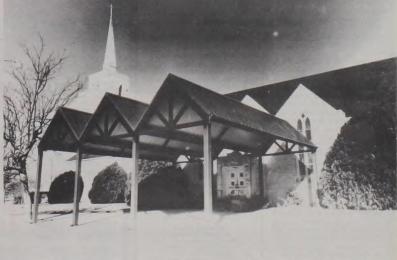
NEARING COMPLETION is the wide, paved drive-through under the protective, steel canopy at the south side door to Sacred Heart Church. Eight steel supports await brick work. Janie Hartman Photo
