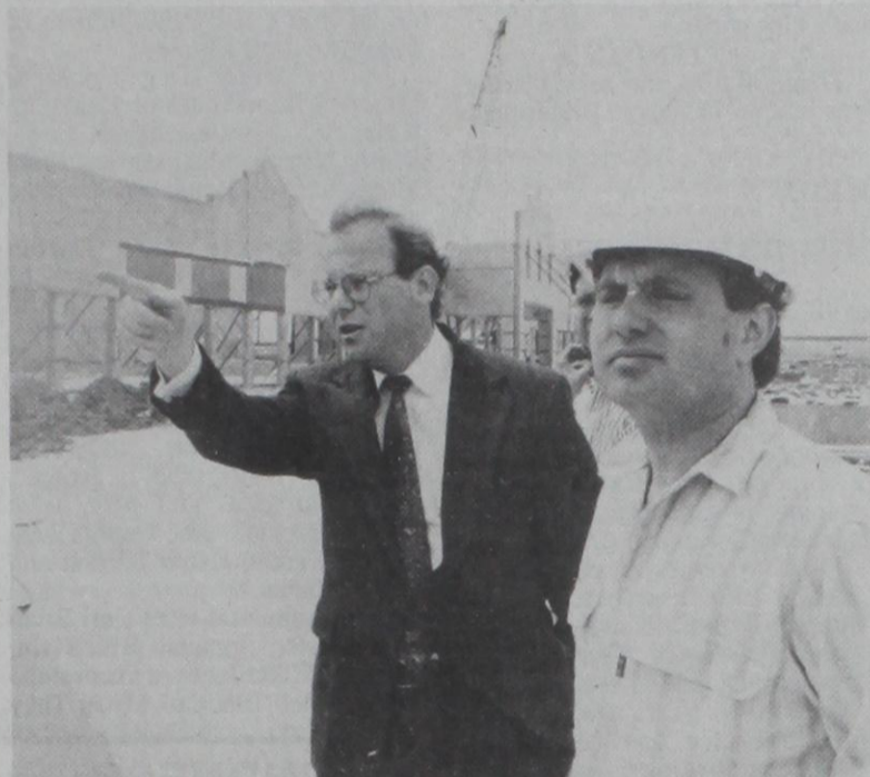
ABRAHAM ROSENTHAL, vice president of the Prime Group of Chicago, Illinois, points to a location on the site of the Gainesville Factory Shops as he explains construction progress. The walls of the retail mall are in the background. The mall will open Aug. 14 north of Gainesville. Elaine Schad Photo
