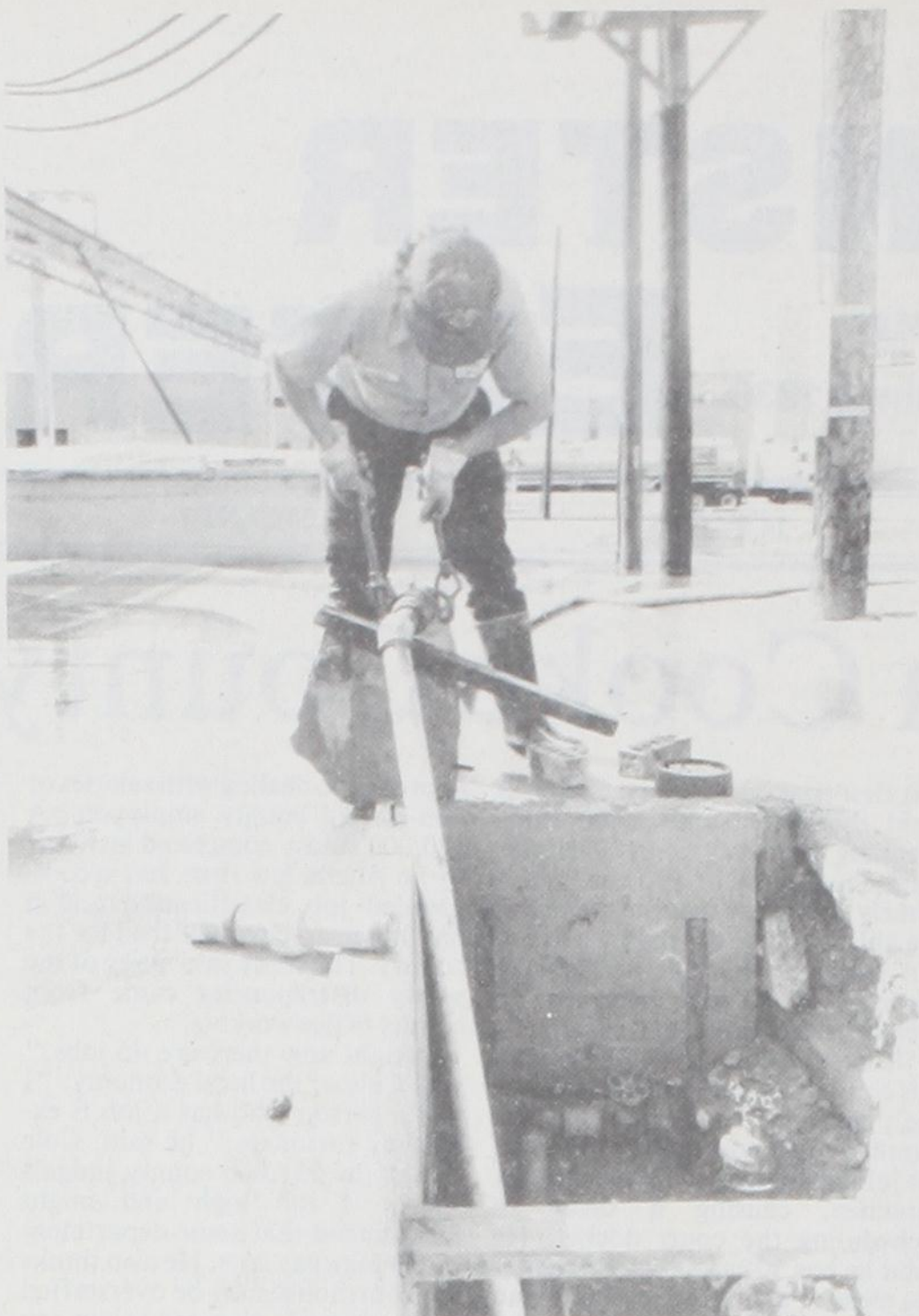
CITY OF MUEENSTER employees took on the job of replacing an 8-inch gate valve on a main water line Monday. The work required turning off the water to AMPI, so a temporary water supply was set up by laying a 2½-inch fire hose from the hydrant at First and Main to the plant's water meter, so AMPI's water input would not be interrupted. In the above photo, Chris Yosten hooks the fire hose to AMPI's water line. Below, David Dittfurth digs away dirt from the 8" valve to be removed on the corner of First and Elm Streets. Janie Hartman Photos
