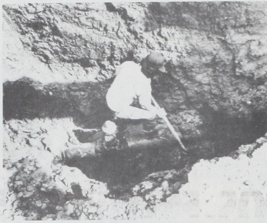
CITY OF MUEENSTER employees took on the job of replacing an 8-inch gate valve on a main water line Monday. The work required turning off the water to AMPI, so a temporary water supply was set up by laying a 2½-inch fire hose from the hydrant at First and Main to the plant's water meter, so AMPI's water input would not be interrupted. In the above photo, Chris Yosten hooks the fire hose to AMPI's water line. Below, David Dittfurth digs away dirt from the 8" valve to be removed on the corner of First and Elm Streets. Janie Hartman Photos
