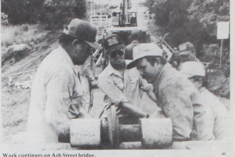
Work continues on Ash Street bridge.
