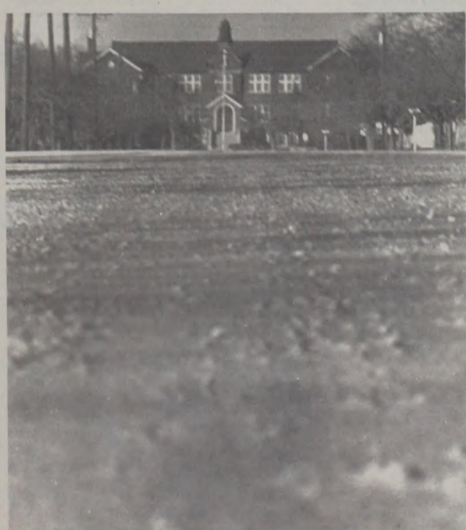
The rough surface of Oak Street is gradually wearing away and contributing to the dust problem experienced by many Muenster residents. Although the current excess gravel will be picked up, next summer's heat will soften the asphalt layer and make a new layer of crushed rock probable. Staff Photo
