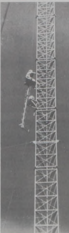
A WORKER helps lift an antenna that will be used by AgComm, up the newly-installed tower located east of Muenster on the Cooke County Electric Co-op grounds. The new tower replaces the one blown down last spring north of town and will presently hold two antennas. Janie Hartman Photo
