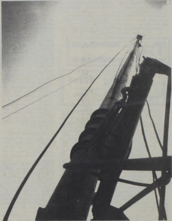
As large dark clouds teasingly pass overhead, this rig at the Tony Rohmer home is being used to help in the present
