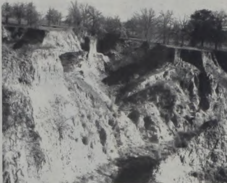
The gullied area pictured above is to be shaped, vegetated, and stabilized with a grade stabilization structure. This area northeast of Alvord, is to be reclaimed as part of the Big Sandy Creek Watershed plan.
