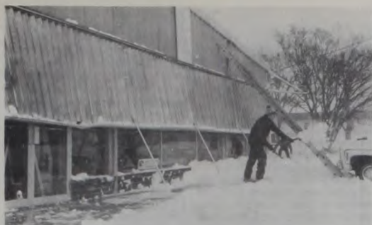
THE SNOW was light and powdery, but the accumulated weight was enough to collapse the awning at Hennigan Auto Parts. Janie Hartman Photo
