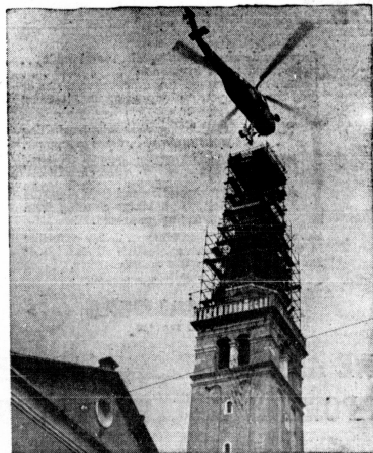
CLOSER TO HEAVEN —A 600-pound bronze angel is gently lowered into place atop the 16th century church tower of Sacile, Italy, by a U.S. Army "Choctaw" helicopter from the Southern European Task Force. The angel's wooden predecessor was destroyed by quake and wartime bombardment.
