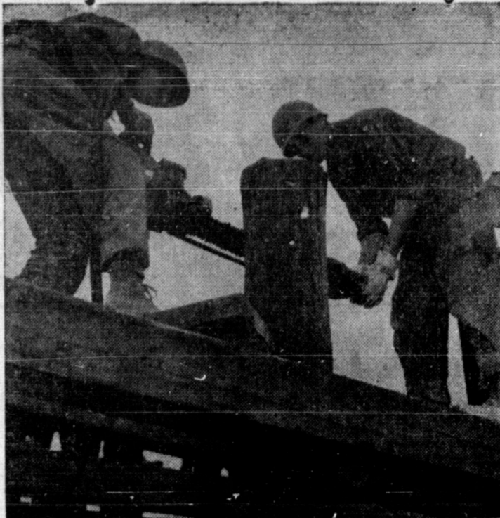
COMBAT ENGINEERS—Two Army reservists from a Minot, N.D., engineer battalion keep in trim for combat engineer duties as they operate a power saw during construction of a bridge across a ravine. They are among 7000 National Guard and Reserve soldiers who went to Fort Carson, Colo., for two weeks of summer training.
