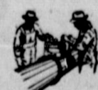
An electronic detector finds the tiniest of flaws in the covering, and these spots are coated by hand.
