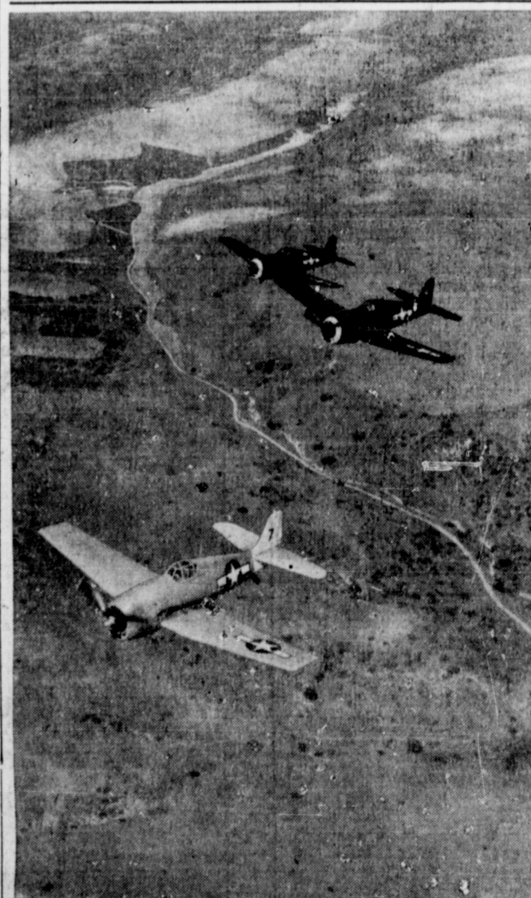
Trailed by two "mother" planes, a pilotless Navy Hellcat (Grumman F6F) soars over the San Diego area in a dress rehearsal for similar air data operations planned as part of the atomic bomb tests at Bikini atoll this summer. The drone (foreground) is controlled by the "mother" Hellcat immediately in the rear while a second plane serves as standby should the first one fail. During the tests four drones, each with two control planes, will be launched from the USS Shangri-la and will be controlled first from the carrier's deck then from a mother plane in the air and finally from the ground controller on Eniwetok where they will land. (Joint Army-Navy Task Force Photo.)
