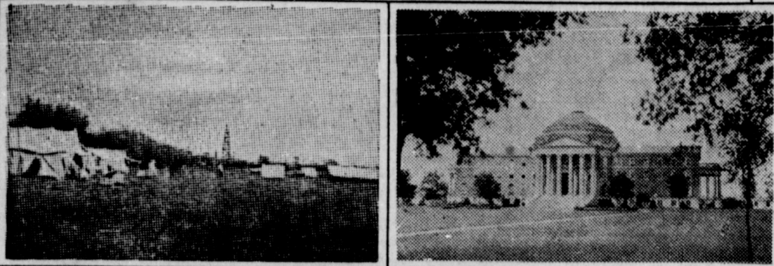
S.M.U. CAMPUS, 1914 CAMP FOR CONSTRUCTION OF DALLAS HALL
