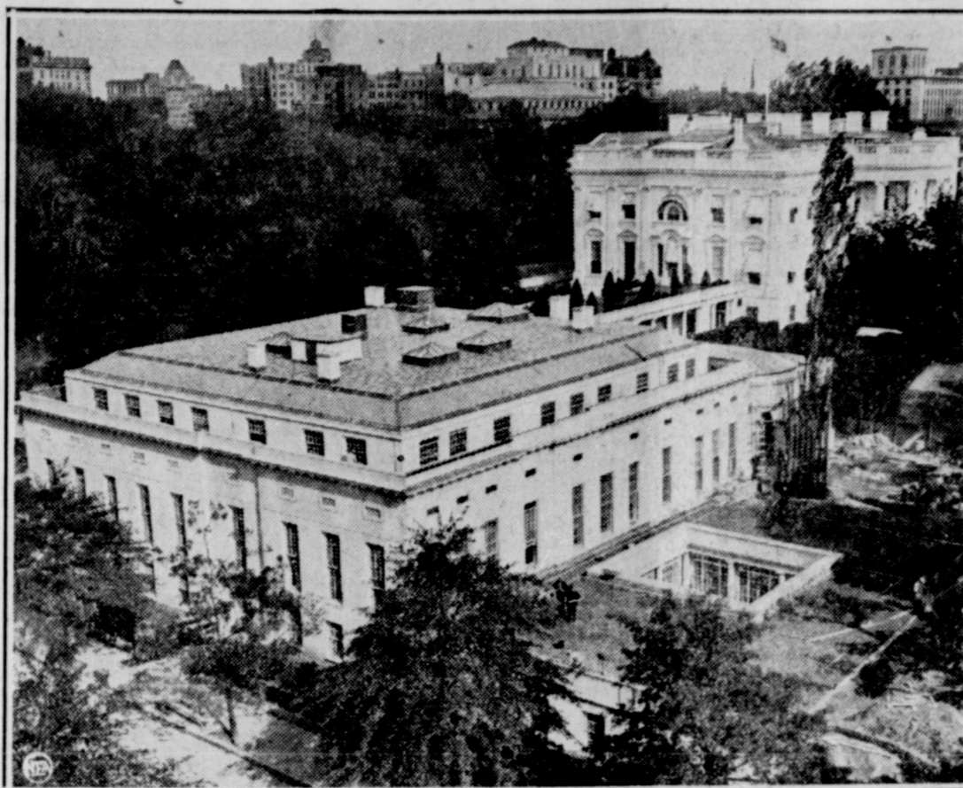
President Roosevelt soon will enjoy a new deal in office space. The enlargement and modernization of the Executive Office building on the White House grounds in Washington, D. C., are now nearly completed. How nearly ready for its occupancy it is can be judged from exterior of the building in the foreground. The roof has been raised to provide an extra floor of offices and extensions have further enlarged the building. In the background is the White House.
