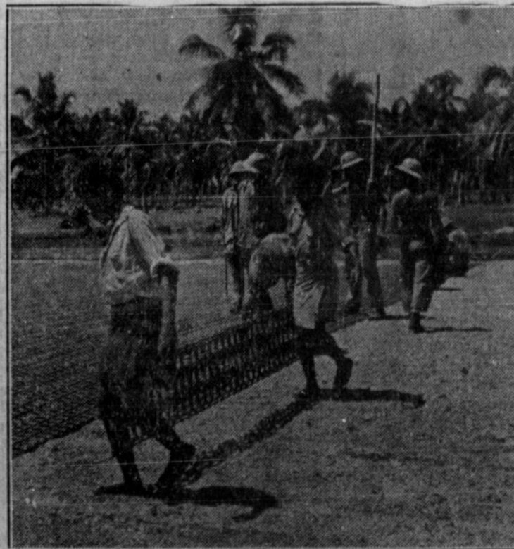
Bureau of Public Relations, U. S. War Department JUNGLE AIR FIELD IN SOUTHWEST PACIFIC —Utilizing native materials and labor, U. S. Aviation Engineers have carved a mile-long runway out of the heart of the jungle. Natives are shown laying the portable steel landing mat under the direction of the Engineers. The foundation is a bed of crushed coral which is locally available in plentiful quantities.
