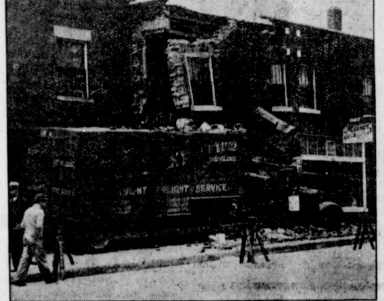
Kansas City, Kans.—A 15-ton wall will not collapse. Such destruction of property, particularly by irresponsible itinerant truckers, is the reason why safety councils nationwide are seeking more stringent laws thoroughly regulating motor transports.
