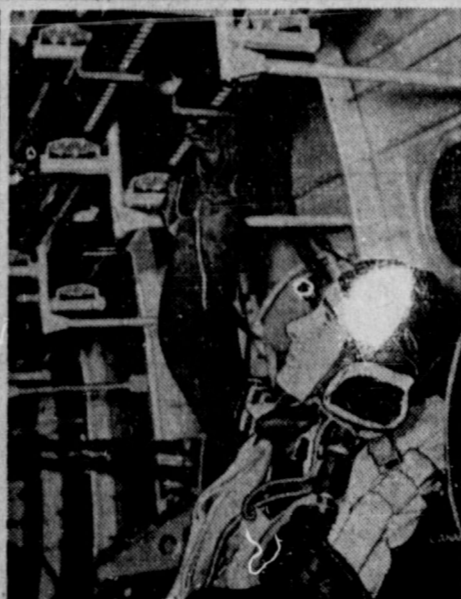
A streamlined conveyor system feeds ammunition to the multiple guns of a Halifax. Before the take-off one of the gunners checks to ensure that there will be no jam in a tight spot.
