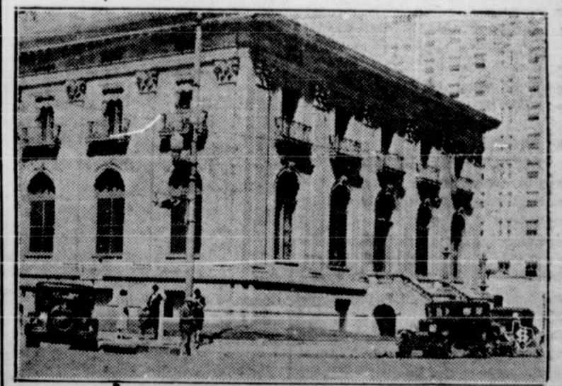
Here is the Federal building at Port Arthur, Texas, from which 1128 pints of choice imported liquor were recently stolen from the U. S. storeroom in the basement, where custom officials had placed it after seizing it from rum running vessels. The thefts were made a little at a time over a period of three months. Five negroes, one of them a janitor of the building, and one white night clerk at the postoffice were arrested.
