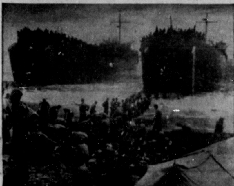
Two Coast Guard men LST's open their great jaws in the surf as soldiers build sanding piers out to the ramps to speed unloading operations on a Pacific Island beach. Some soldiers fill the bags on shore as others form lines and move the bags into place. The supplies and fighting equipment for MacArthur's liberators are bought with your War Bond money. From U. S. Treasury
