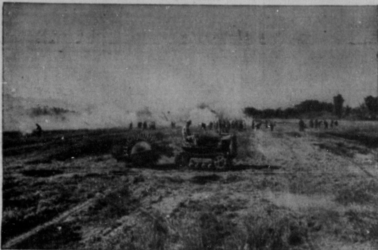
U. S. Signal Corps Photo A U. S. soldier operates an American tractor and sheepfoot roller, smoothing filled ditches on a field being prepared as a C-47 strip. Coolies are cutting and burning grass in the background. Your purchase of War Bonds.
