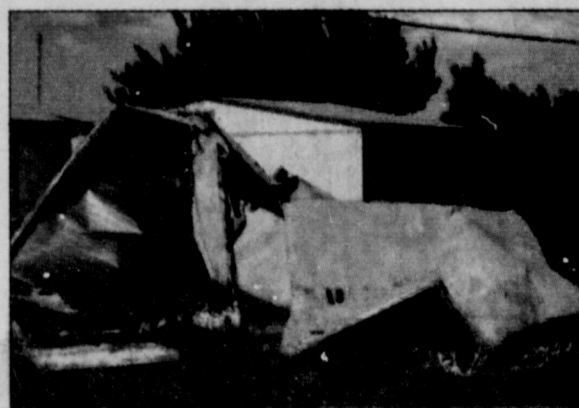
The roof of D.W. Rankins' trailer house landed in a crumpled wreck several feet away, partially crushing a neighbor's chainlink fence.
