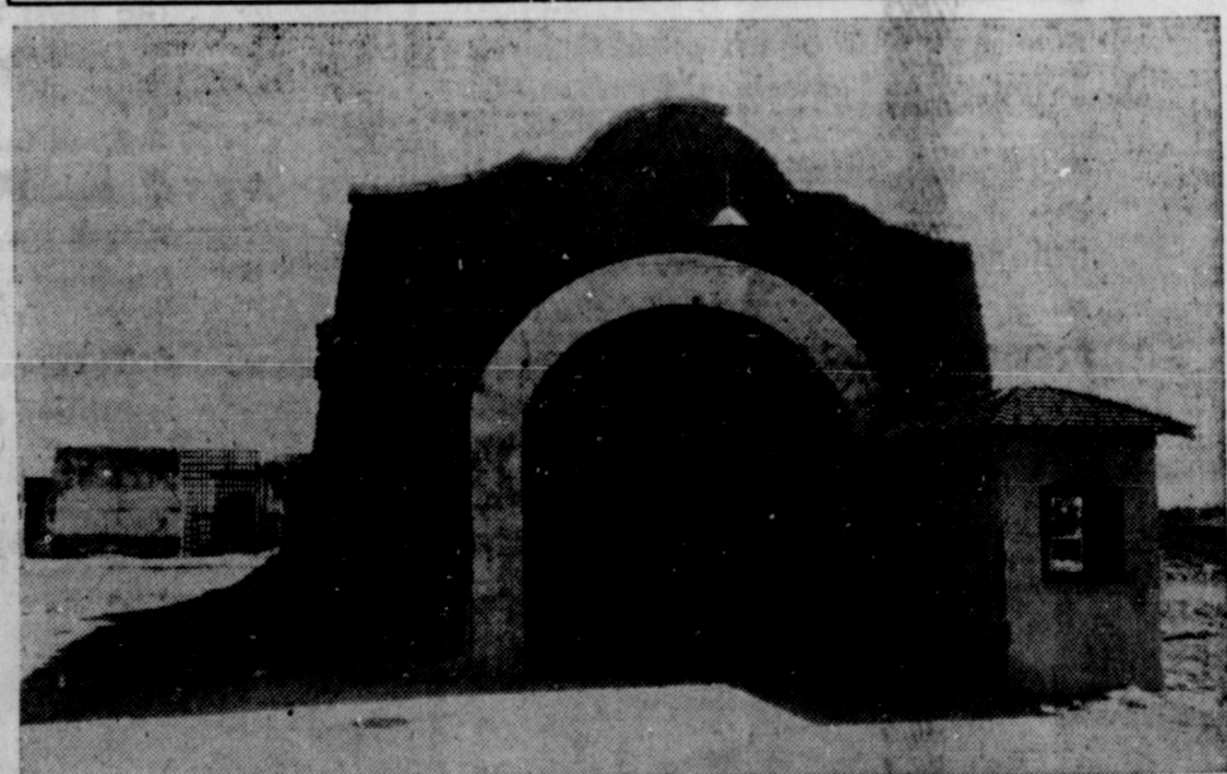
Abandoned in 1909 Arizona's old territorial prison at Yuma has now been taken over by the City of Yuma and is rapidly becoming a focal point for thousands of visitors each year who are shown through the cell blocks and buildings which once housed many of Arizona's most dangerous bad men of pioneer days.
