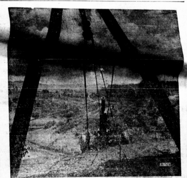
NECESSITY THE MOTHER OF INVENTION—A 105mm howitzer of the 2d Howitzer Battalion, 9th Artillery, 25th Infantry Division, reaches the crest of an almost perpendicular slope in the Koolau Mountains of Hawaii after being hauled up by engineers using an ingenious arrangement of ropes, an A-frame and manpower. It's part of the training of one of the units selected for duty in Thailand.
