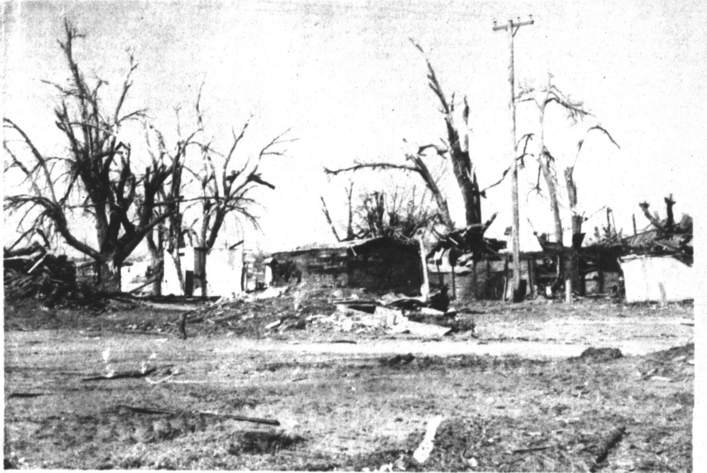
Residents of Lefors were in the midst of a huge clean-up campaign earlier this week, using every means to clean off lots so that new buildings can be constructed in the wake of last Thursday morning's tornado. Residents are in need of funds to build back homes and businesses destroyed by the storm.
