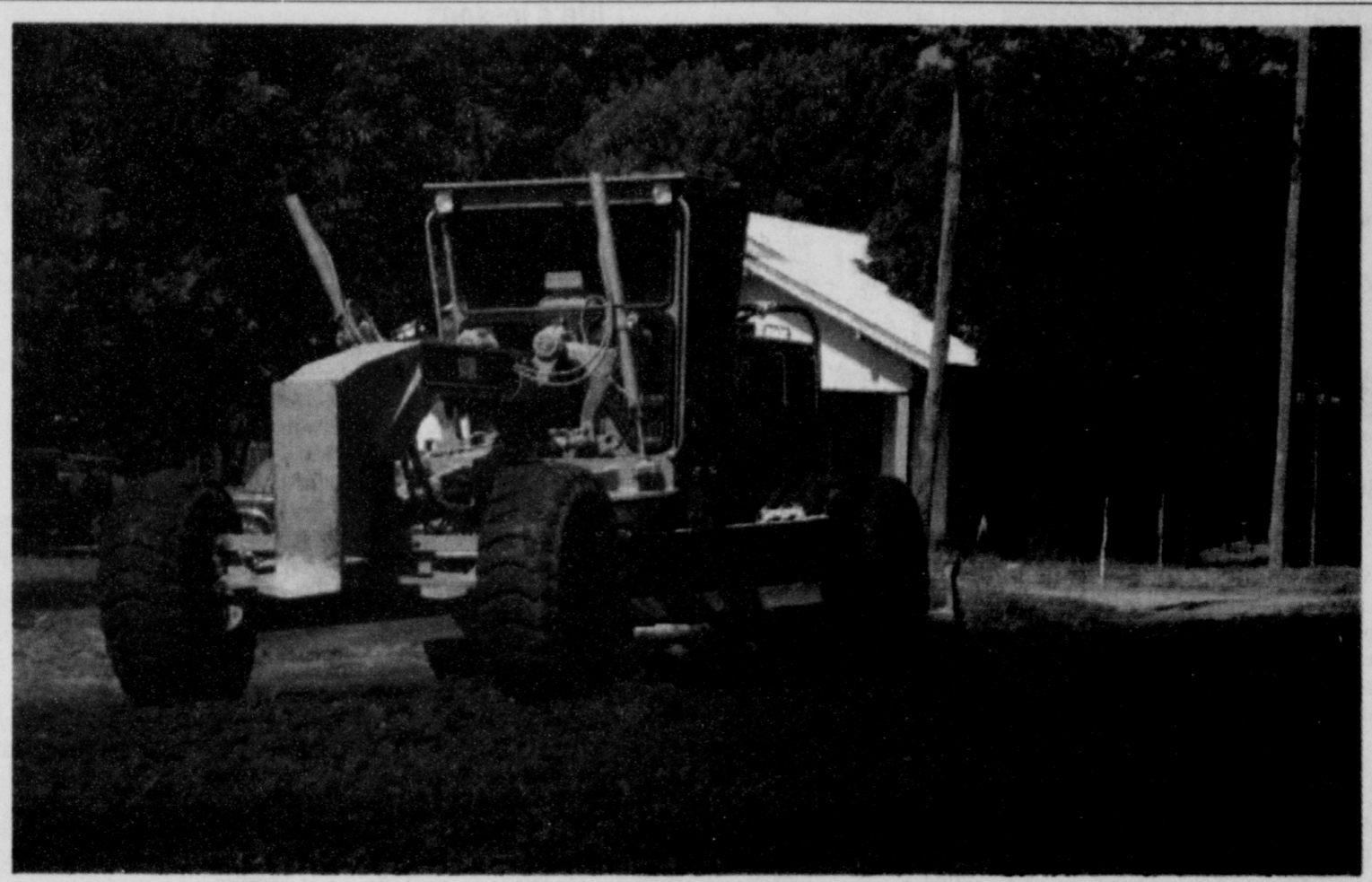
B&B Solvent began work on West Sixth Street between Cottage and Collinson this week as part of a 60-block paving project. Enterprise photo
