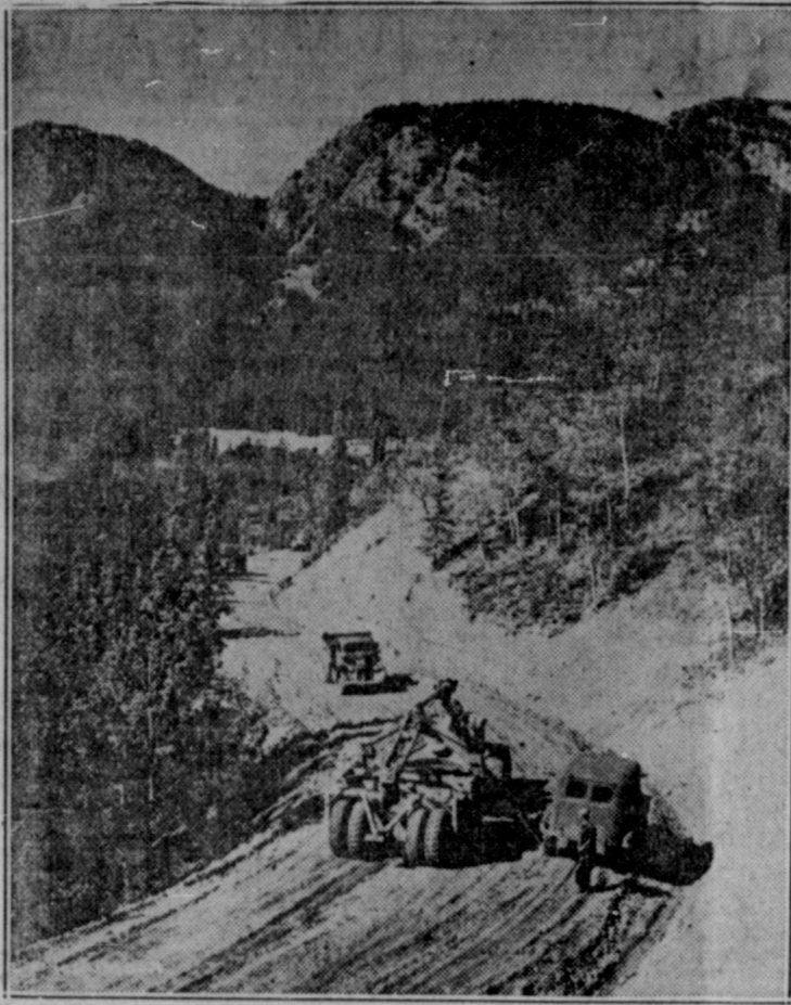
By Bureau of Public Relations, U. S. War Dept., Wash., D. C. ALCAN HIGHWAY UNDER CONSTRUCTION—In the fastnesses of Alaska's mountains the "carry-all" puts the finishing touches on the gravel surface of the great road.
