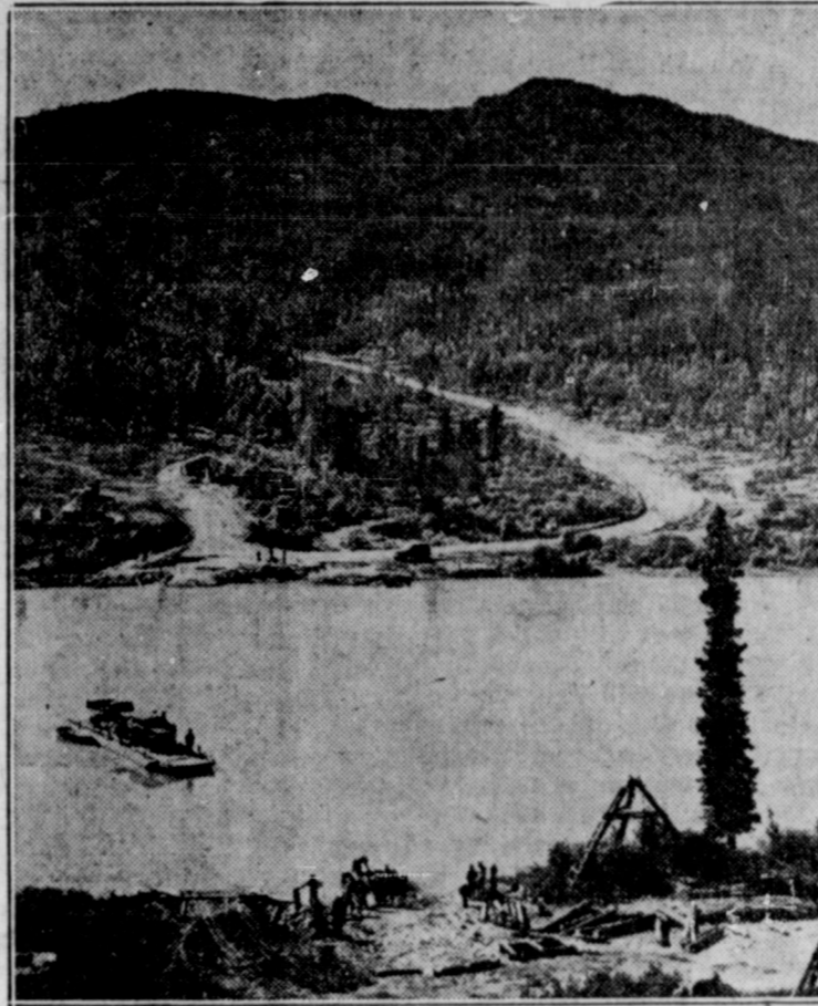
By Bureau of Public Relations, U. S. War Dept., Wash., D. C. ROPE FERRY ON ALCAN HIGHWAY —A typical engineer ferry utilizing the speed of the current to force the boat across by the use of a wire cable stretched from shore to shore.
