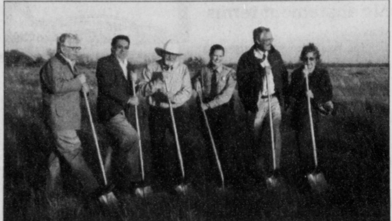
Caprock Canyons State Park dignitaries break ground for a new visitors center last week.
