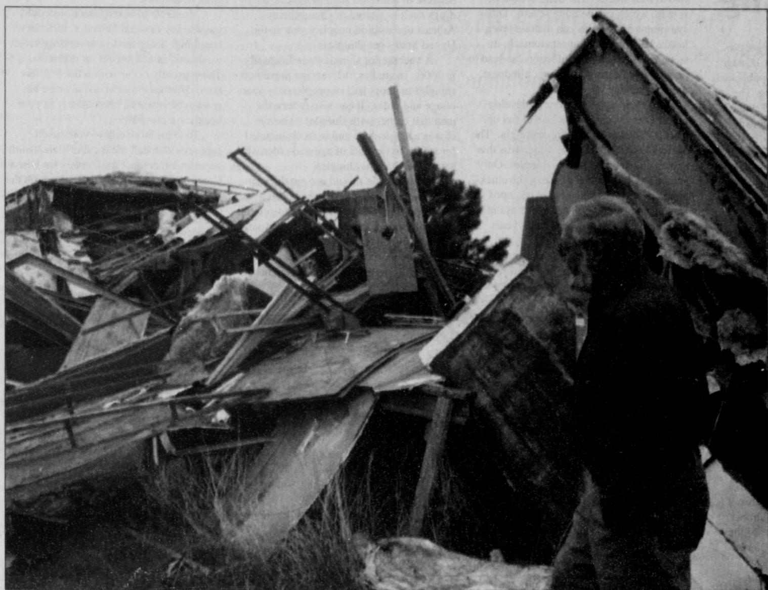
James Homer surveys the damage from a Saturday storm to a mobile home he was using for storage.
