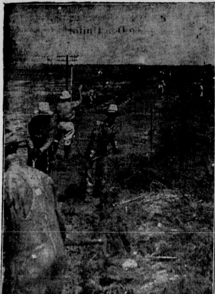
Scenes of the disastrous Lelia Lake flood bring to memory one of the heaviest rains in this section in 10 year's time. Three lives were lost and thousands of acres of crops completely destroyed by the rushing water. The picture at left shows workers rebuilding Fort Worth & Denver tracks near Lelia Lake, and at right, a trestle on the railroad near Wellington was washed out completely, leaving only the rains spanning the gap. —The Clarendon News, June 16, 1938.
