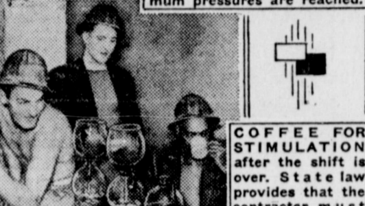
COFFEE FOR STIMULATION after the shift is over. State law provides that the contractor must provide coffee free of charge when men return from the compression locks.
