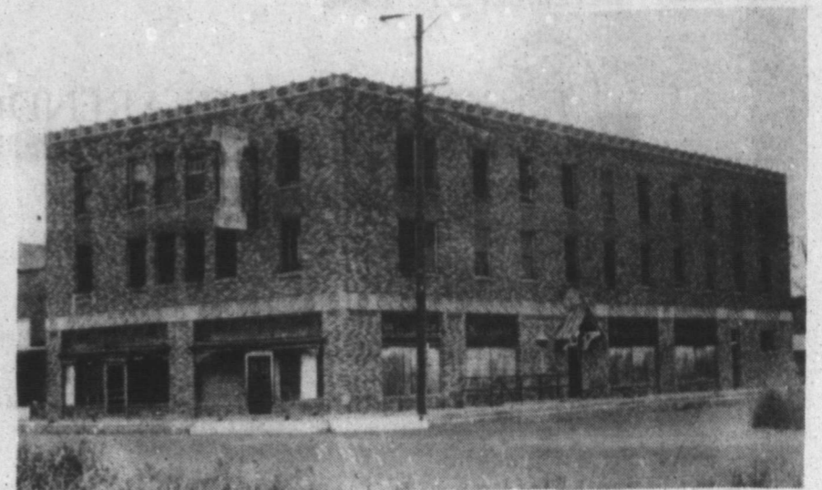
OLD ANTROBUS HOTEL in Clarendon, Texas in 1992. Windows are boarded up and are missing. You can clearly see the tin shingles that now reside in Plano.
