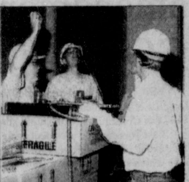
Project manager Stephen Dodge, architect John Volz, and electrician Ben Cherry discuss lighting in the J.P. office.
