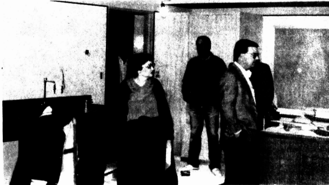
CLARENDON SCHOOL BOARD MEMBERS Venita Sharrar, Todd Knorpp and Fred Clifford inspect the construction of the new High School building.
