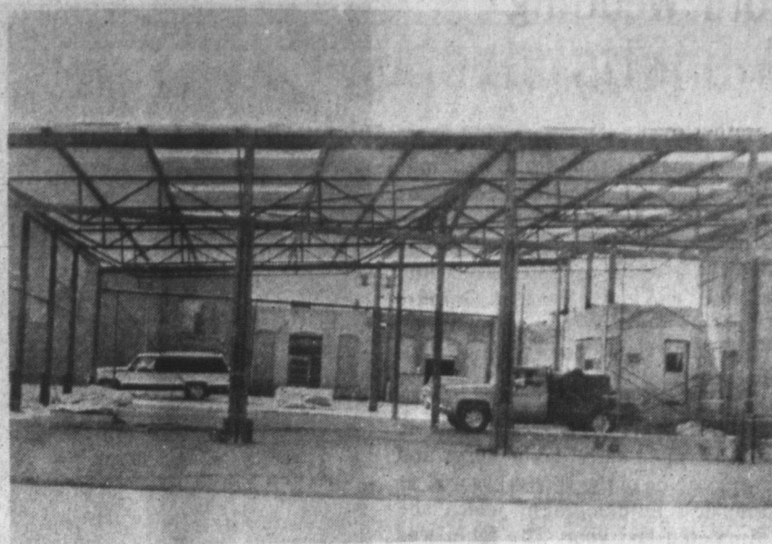
CONSTRUCTION OF FIRE STATION ADDITION
