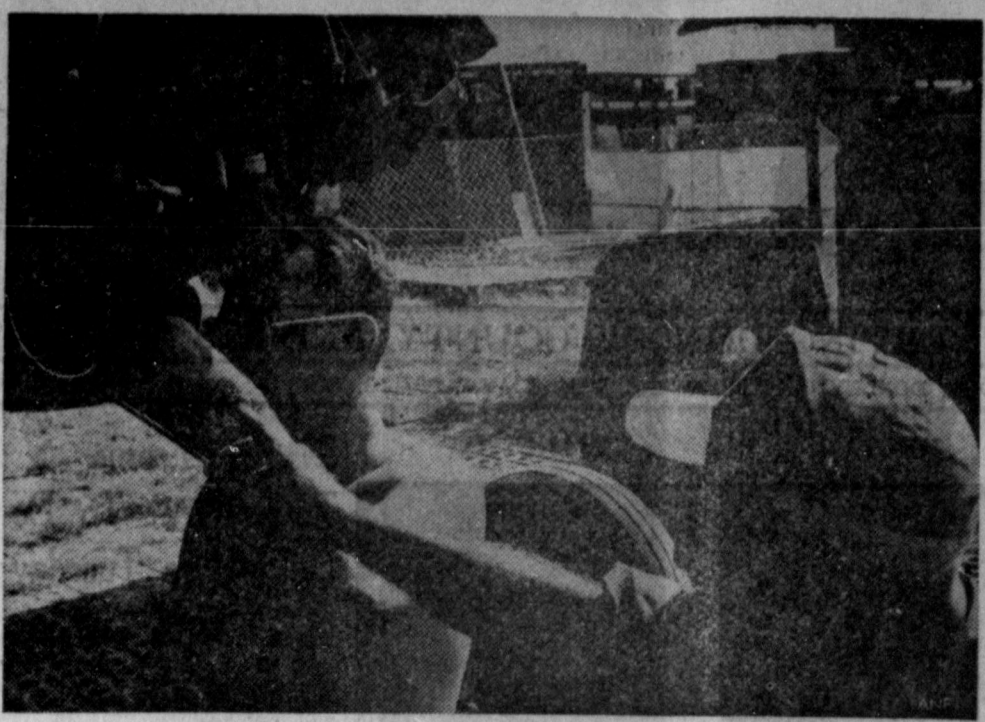
CLOSE SCRUTINY — Sp5 William L. Crowl (left) and Sfc. Richard L. Ovelman service the engine of a BEAVER utility airplane. Specialist Crowl, Boonsboro, Md., and Sergeant Ovelman, Hagerstown, Md., are both members of the Army Reserve serving with the 357th Transportation Company (Aircraft Maintenance Direct Support). The Pennsylvania Reserve unit, called to active duty last April, has the mission of maintaining helicopters and fixed-wing aircraft at Bien Hoa Air Base, Republic of Vietnam.
