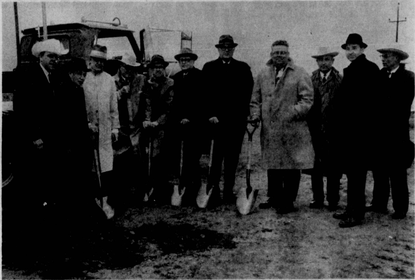
GROUND BREAKING FOR THE NEW LAKE--It was a cold April afternoon in 1966 when this group gathered at the site of the new Lake Greenbelt north of Clarendon for official ground breaking ceremonies. Shown here left to right are Senator Andy Rogers, Clifford Johnson, Greenbelt directors; Howard B. Boswell, Austin, and Marvin Shubert, Petersburg, of the Texas Water Development Board; William E. Berger, Texas Water Rights Commission; Dr. S.H. Townsend, president of the Green-
