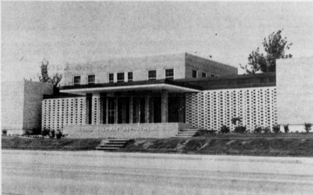
THE NEW HIGHWAY DEPARTMENT district headquarters at Childress completed in recent months is indicative of the importance placed on highway growth in the Greenbelt area. Construction is currently underway on a complete four-lane divided highway along U.S. Highway 287 connecting Quanah, Childress, Memphis, Hedley and Clarendon with both coasts of this nation as well as Mexico and Canada.
