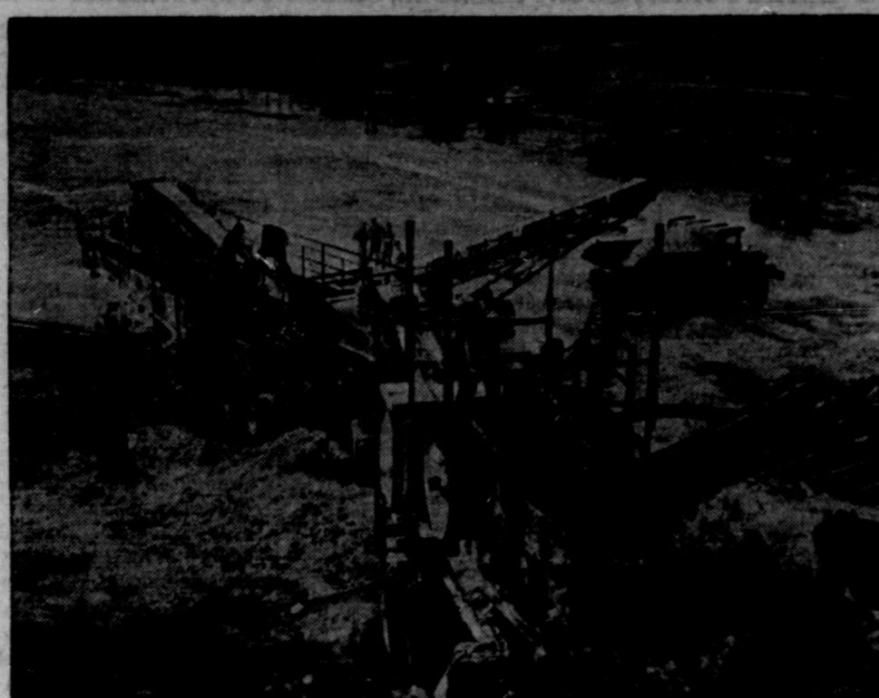
BREAK IT UP! —Army Engineers of the 362d Engineer Company are feeding granite into a 75-ton-per-hour rock crusher in Vietnam. The machine crushes the granite into small pieces for use as an aggregate in concrete mixed for construction projects. Material for the crusher is obtained by drilling and blasting on the side of a two-million cubic yard granite mountain nearby.
