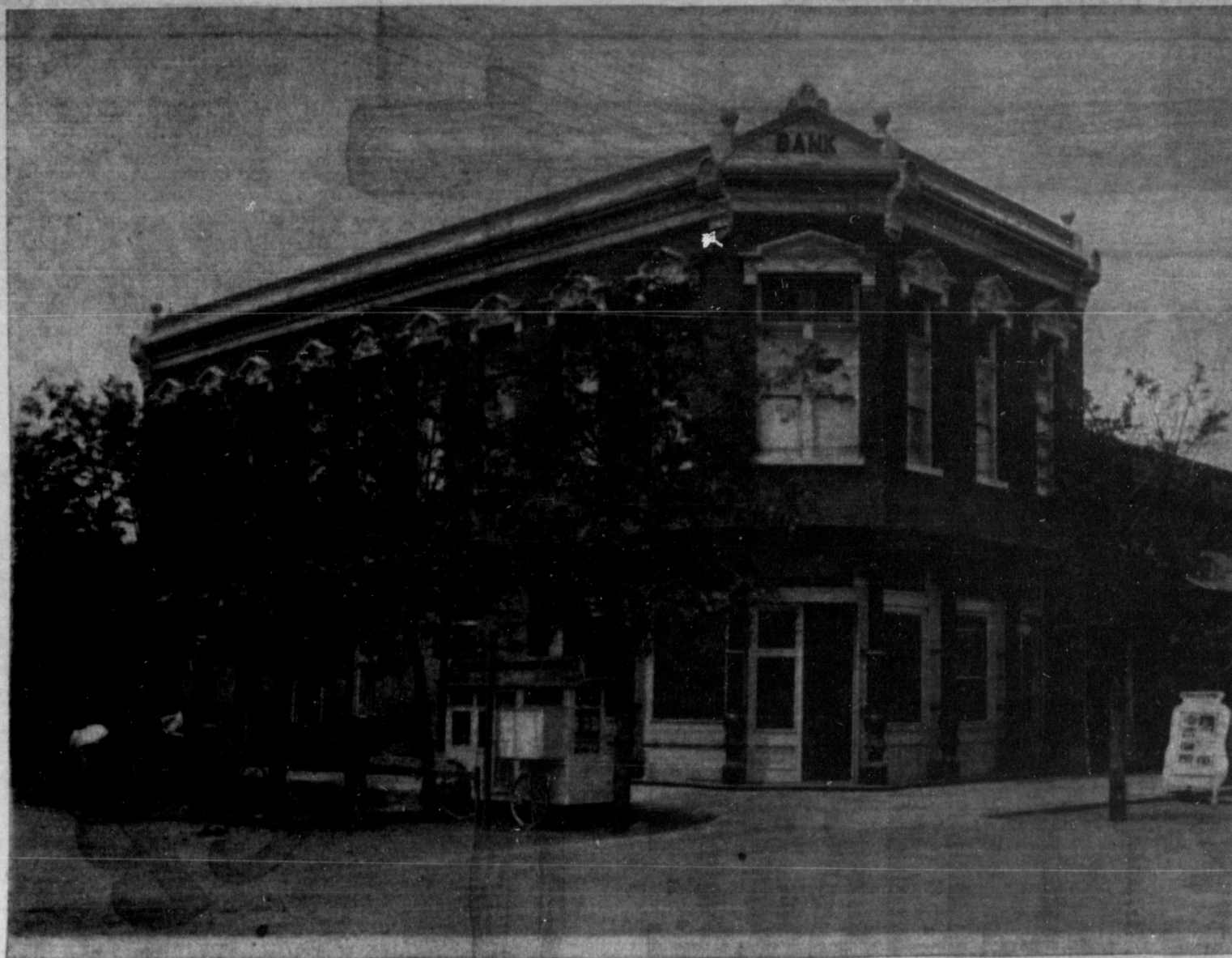
Remember When—This is how main street intersection looked in new Clarendon a few years ago—in the horse and buggy days. This was the First National Bank that was constructed around the turn of the century and only recently, the remodeled version was torn down to make way for the new parking lot at Cliffords' Grocery. New brick now face the south wall of the grocery store and certainly add to the appearance of main street and highway intersection.
