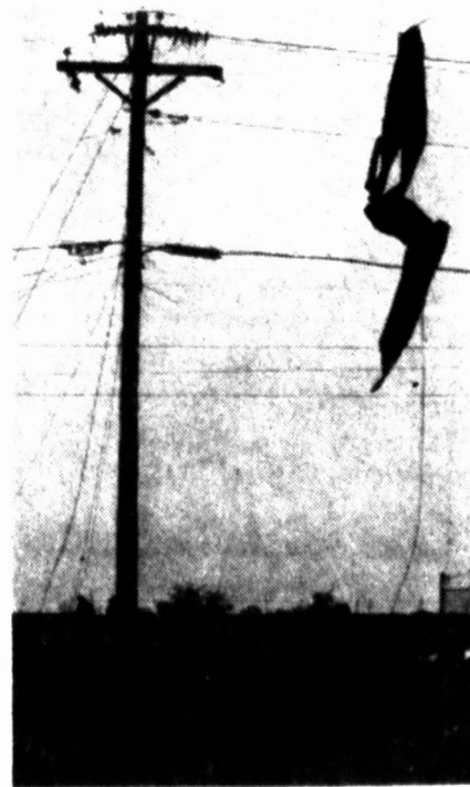
Sheet Metal hanging from power line as a result of the tornado that hit Howardwick Sunday night.
