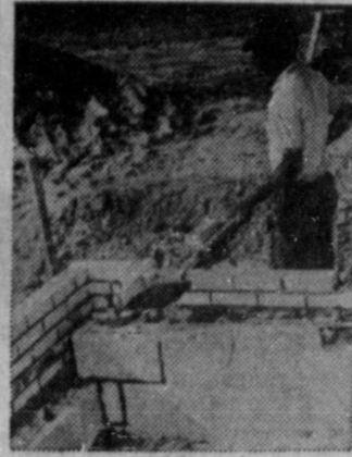
WORKER FILLS the hollow cores of wall blocks with sand to provide added shielding against radiation—one of several techniques used to build low-cost fallout protection into a new church at McLean, Va.
