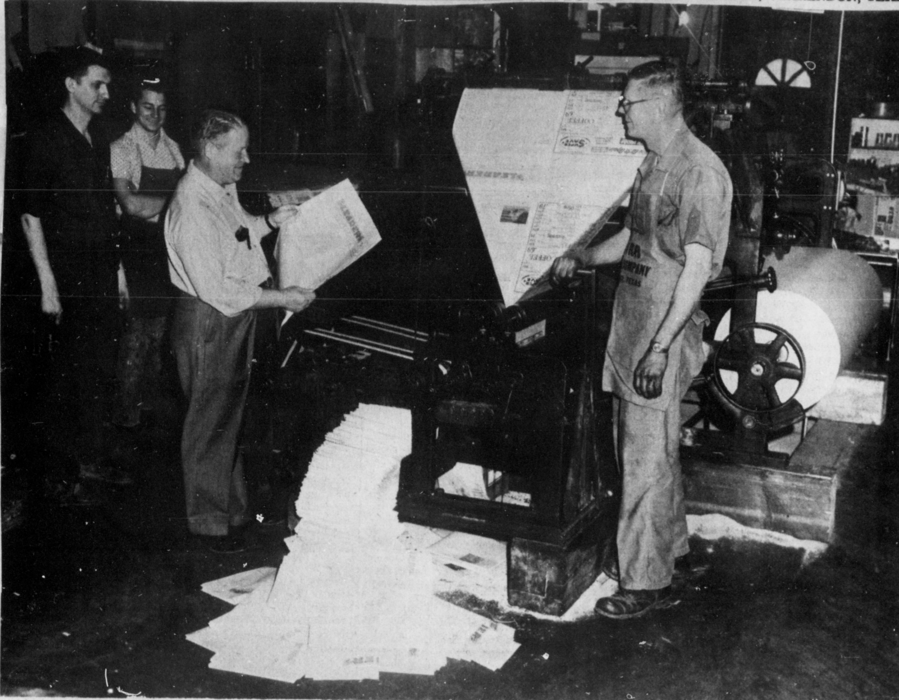
Back in 1968 this Goss Comet roll fed press was installed to print the Leader. This was the first edition off the press. Left to right, Bill Tipton, Ernest Moreland, Editor G. W. Estlack and John Just. Photo by Saye's
